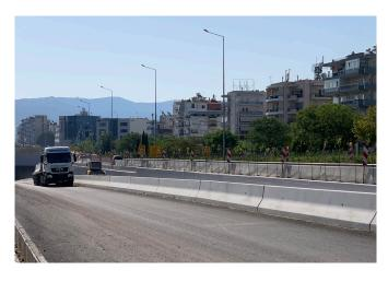
Containment level Working width Impact severity level H2 (covers H1, N1, T3, T2, T1)
