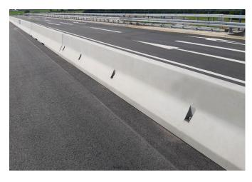
Containment level Working width Impact severity level H2 (covers H1, N1, T3, T2 and T1) W2 (covers W3, W4, W5, W6, W7 and W8)
