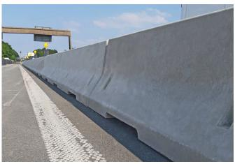
Containment level Working width Impact severity level H2 (covers H1, N1, T3, T2 and T1) W1 (covers W2, W3, W4, W5, W6, W7 and W8) **ASI B**
