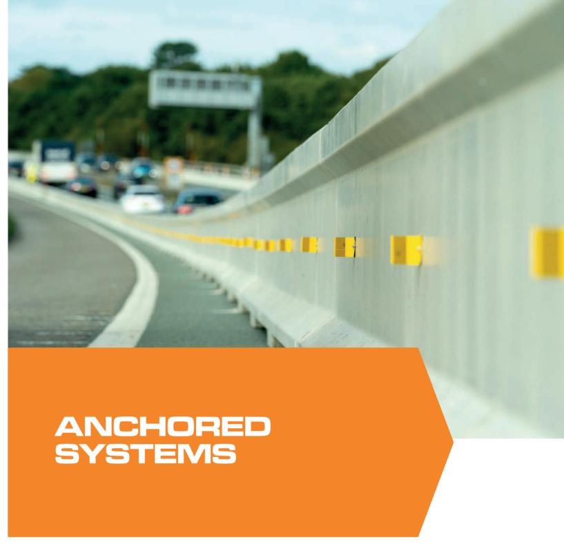
REBLOC anchored barriers can be used as single-sided and double-sided systems for the central reserve and along the verge.
