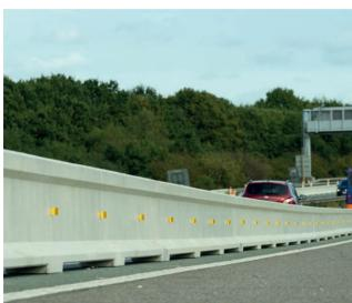
REBLOC RB80SA\_4 and RB80SA\_12 are free-standing precast concrete vehicle restraint systems designed to provide protection on high-speed roads and motorways where space is limited.
