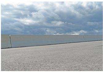
Containment level Working width Impact severity level H2 (covers H1, N1, T3, T2, T1) W2 (covers W3, W4, W5, W6, W7 and W8) ASI B
