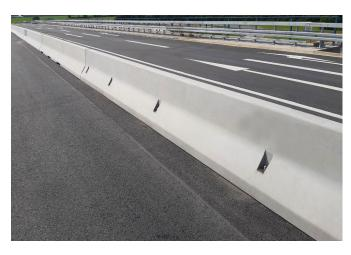
Containment level Working width Impact severity level H2 (covers H1, N1, T3, T2 and T1) W2 (covers W3, W4, W5, W6, W7 and W8)
