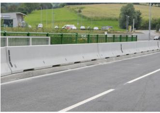
Containment level Working width Impact severity level H2 (covers H1, N1, T3, T2 and T1)
